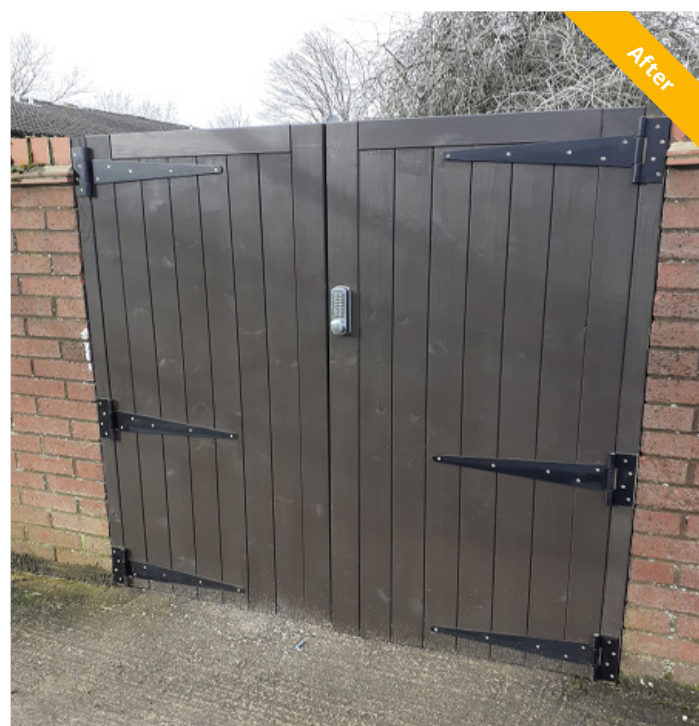
Praetorian Court - gates added to bin stores
