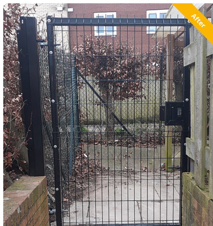
The Close now with the metal gates installed
