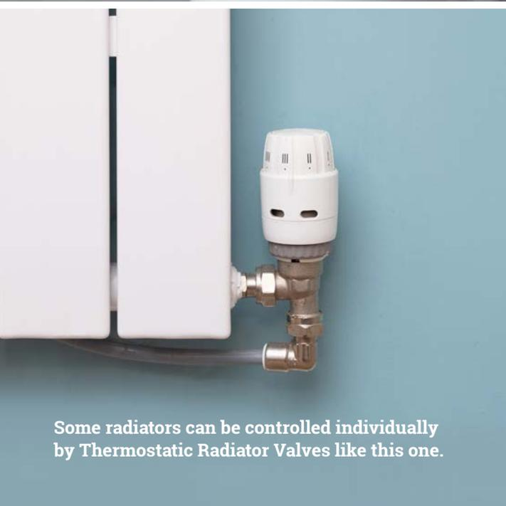
Some radiators can be controlled individually by Thermostatic Radiator Valves like this one.
